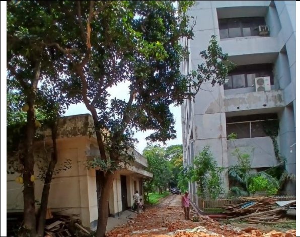
Widening of Entrance Road to the project site during visit on 12.05.2026
