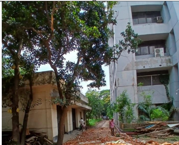
Existing structure (left) will be used as site office after renovation works
