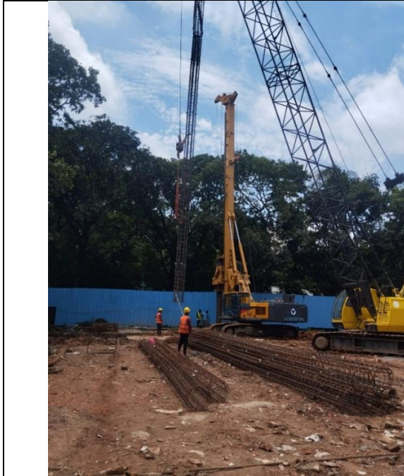
Lowering Rebar Casing inside the Shore pile
