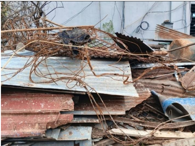
Debris stack pile at the corner of the project site
