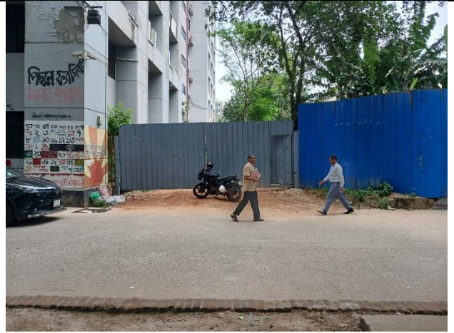
Construction of Entrance Gate date 30.06.2026
