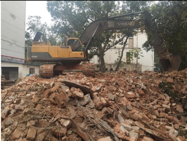
Demolition of existing structures inside the project site. Date of Photograph 12.05.2026
