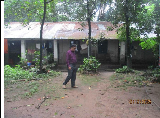
Existing Tin Shad Structures at Proposed Site at DU, Date 13.07.2025
