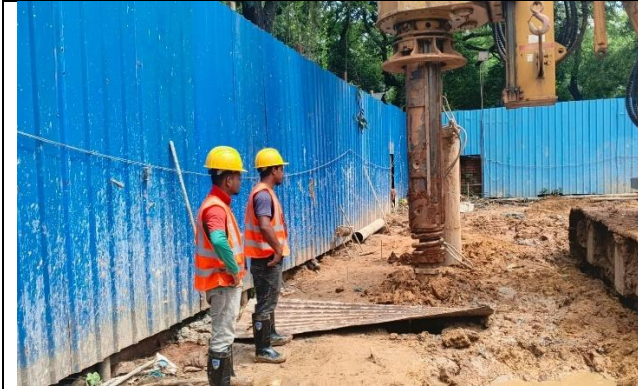
Auger Rotary boring for the Shore piling works
