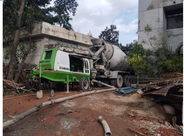
Carrying of Concrete Mixer from the Pre-Mix Batching Plant
